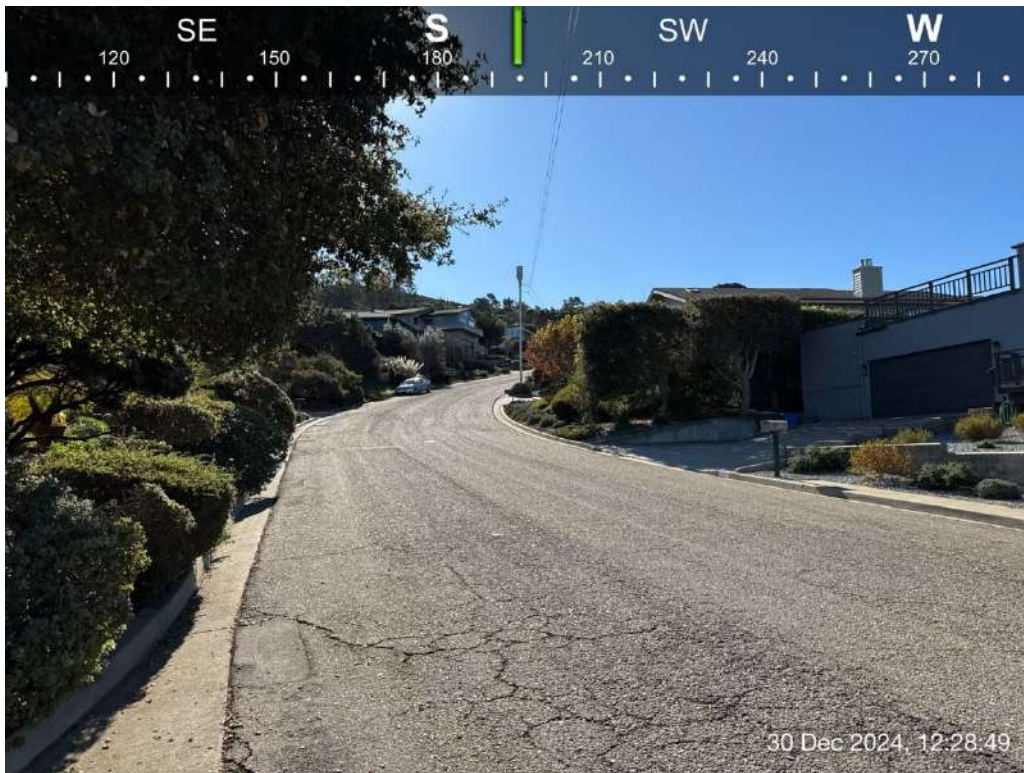
Photograph 26: Travis Drive facing south at Houston Drive.
