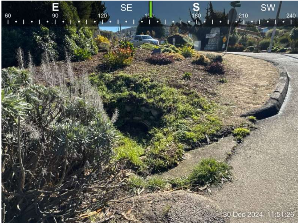
Photograph 17: Drainage culvert along Pecho Valley Road.
