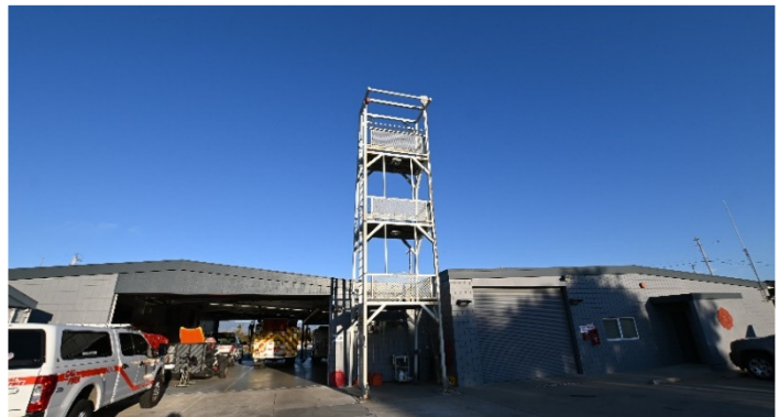
Existing Hose Drying Tower at the back of the Apparatus Bay
